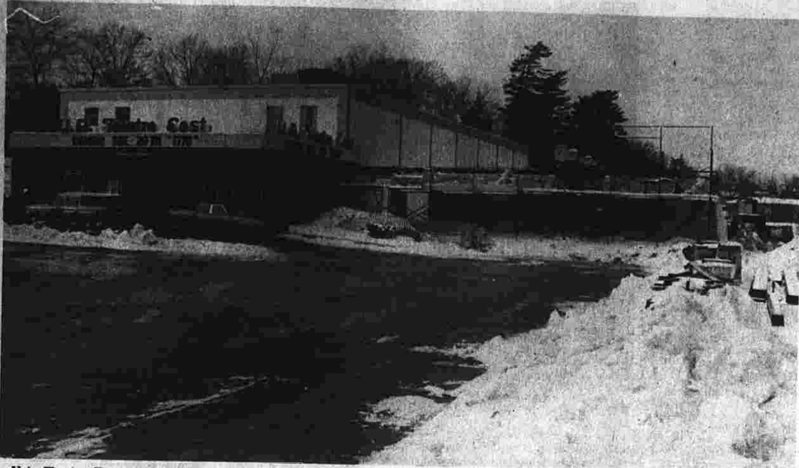
The U.A. Theatre East will soon be having company. Under construction beside the theatre is a smaller twin theatre with a seating capacity of 500 as opposed to the U.A.'s capacity of 800. The new Twin Theatre, also owned by United Artist's, will share a common lobby.
